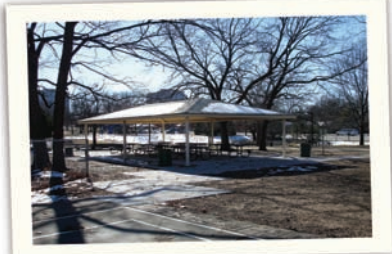
Newly completed LaFortune Park picnic shelter
