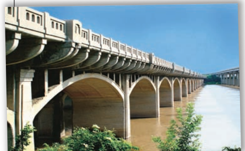
Historic 11th Street Bridge across the Arkansas River
