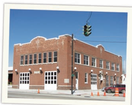
Collinsville City Hall
